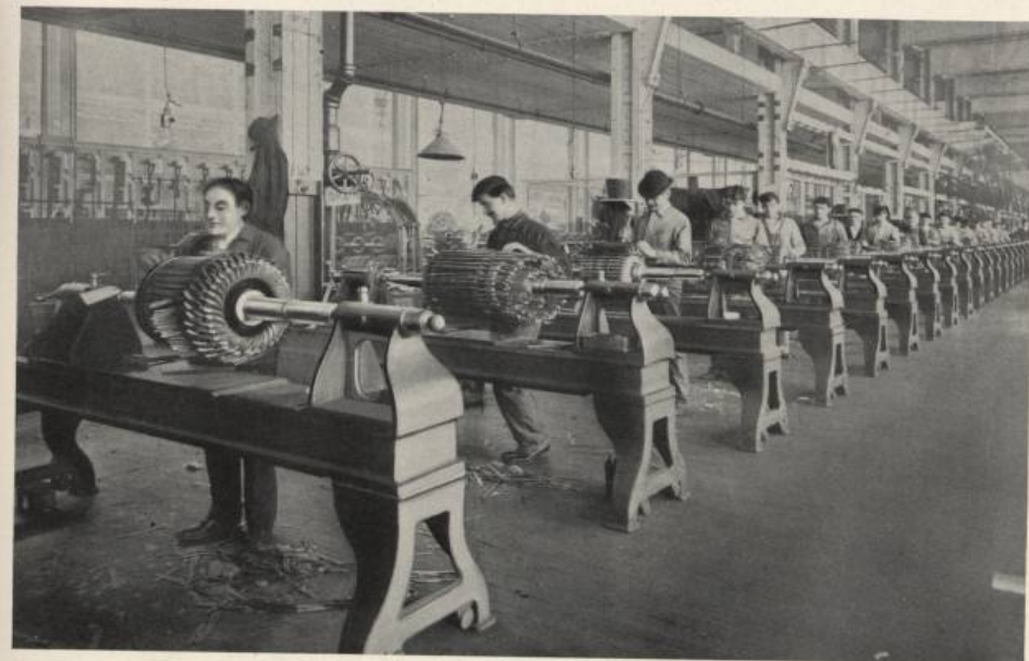
WINDING RAILWAY MOTOR ARMATURES
