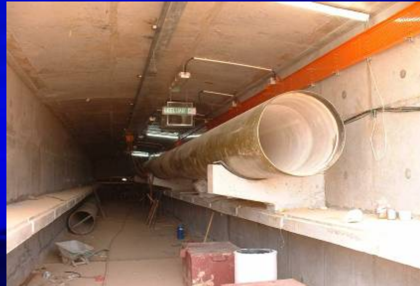
INSTALLATION OF THE 800mm DIAMETER WATER PIPES
