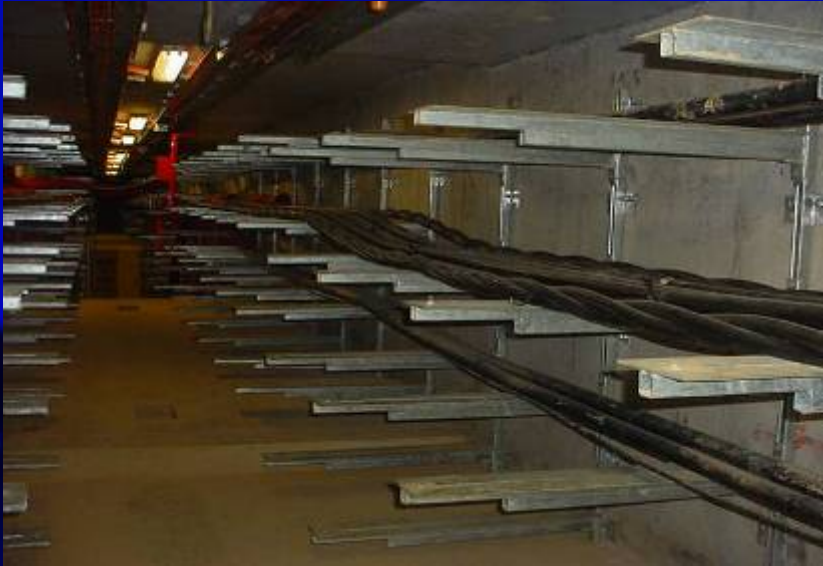
T.N.B CABLES LAID AT THE STANDARD C.U.T SECTION
